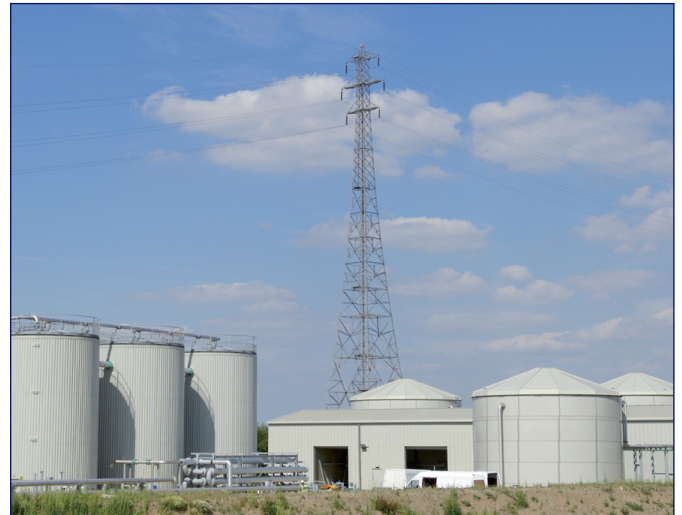
Kings Lynn biosolids treatment works.
